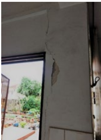
Figura 3. Recalque
